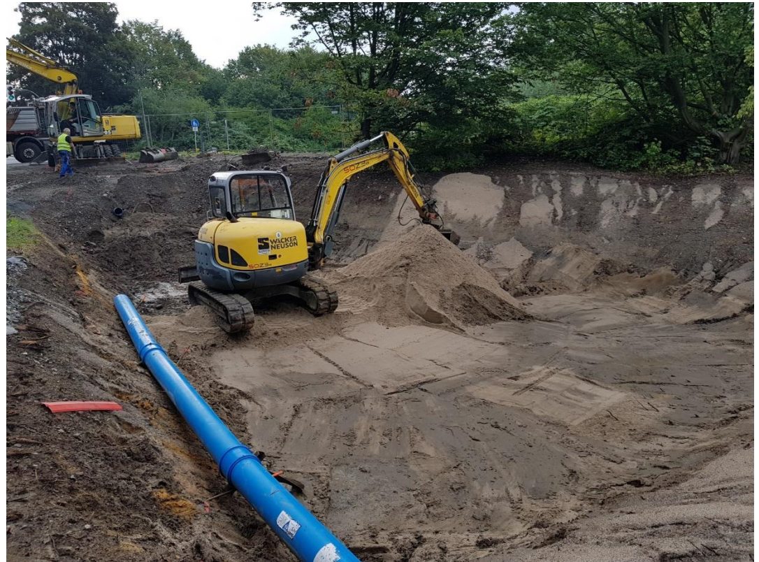
Abb. 15: RRB A = \text{ca. } 145 \text{ m}^2 , V = \text{ca. } 65 \text{ m}^3
